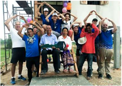
Australia Wooden house for Rom Phoun Siem Reap | July 2-6, 2018
